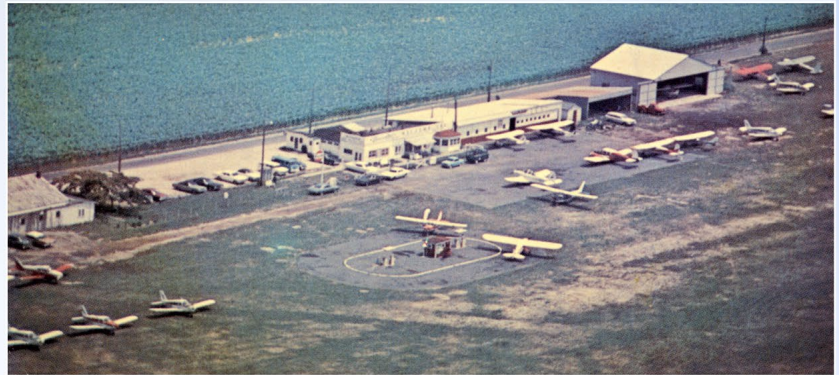
Rehoboth Airport, Rehoboth Beach, Delaware
