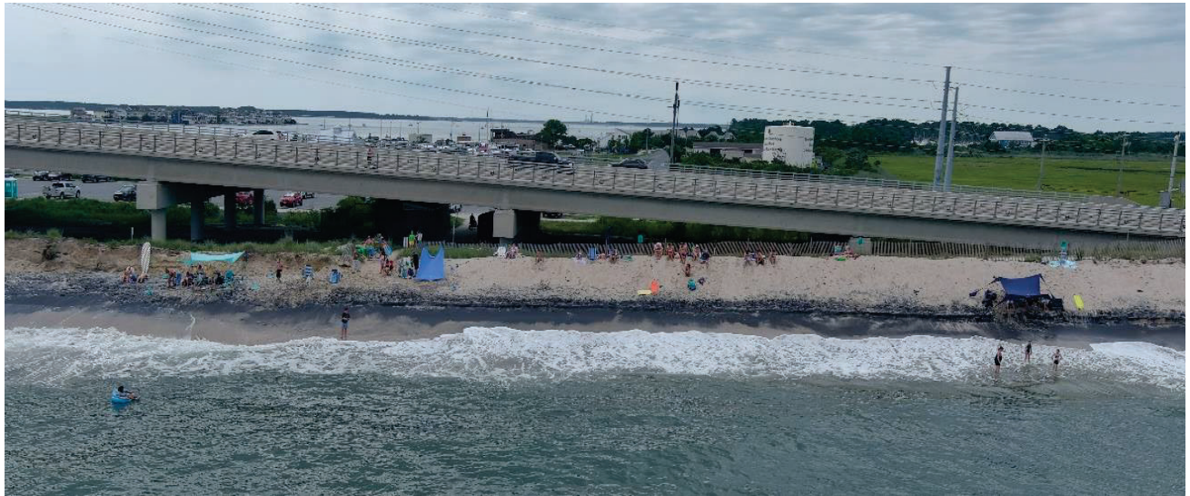
Figure 5. July 26, 2024. View of North Beach from the Atlantic Ocean during high tide. No observable dry beach above the intertidal zone. Beachgoers sit on the dune face and crest.
