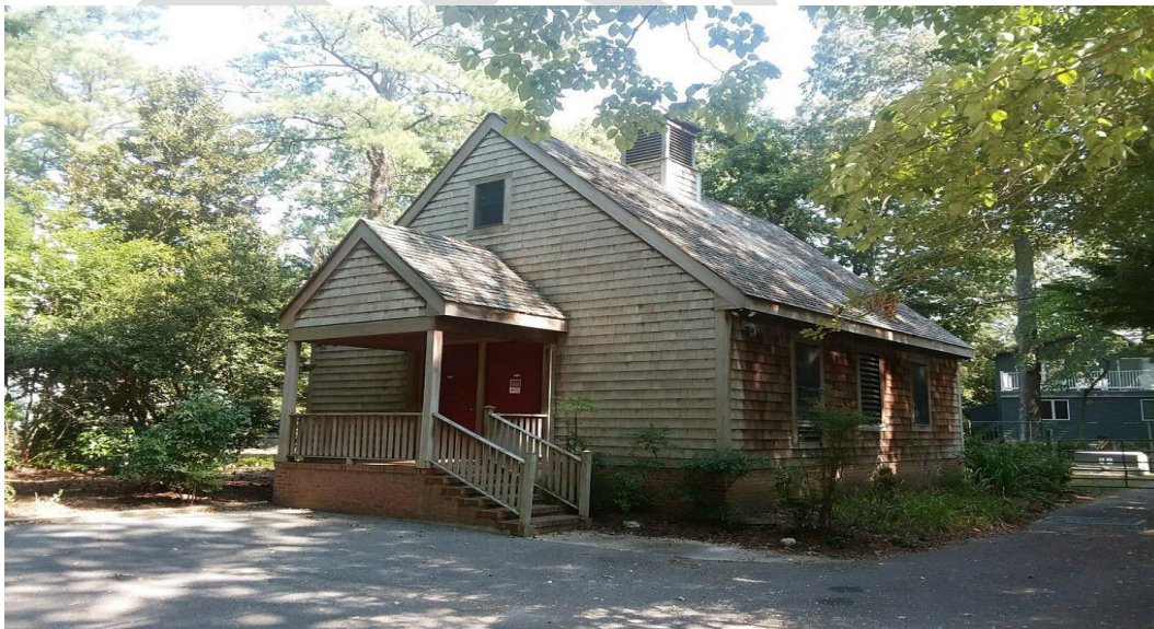
Figure 12. Town Water Plant.
