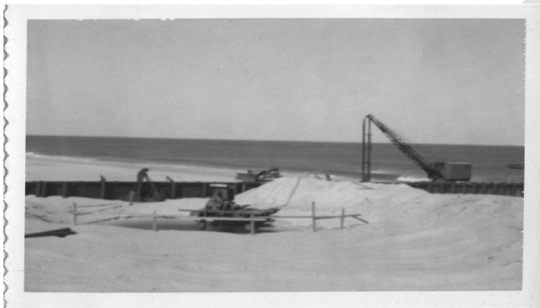
Figure 5. Construction of Jetty – Photo by Wilbur Corkran 1958.
